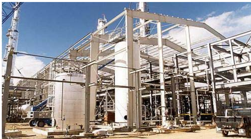
Figure 2. Lost Cabin Gas Plant (shown during construction of enclosing structure).
