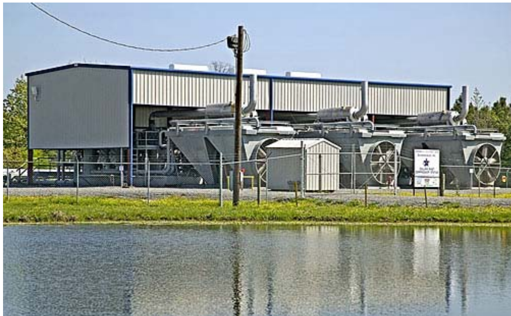
Figure 1. Large Compressor Station (American Central Gas Compressor Station; Carthage, TX).
